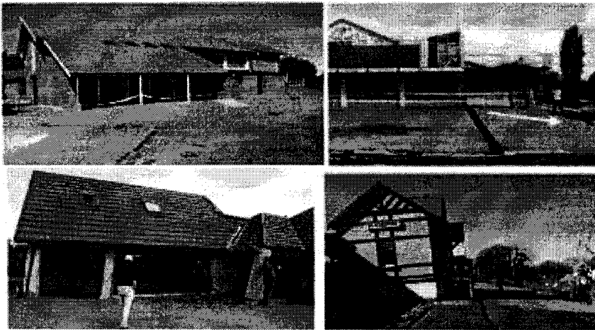
Figure 10 : Views of damage to buildings caused by ground liquefaction during the 2010 earthquake.
