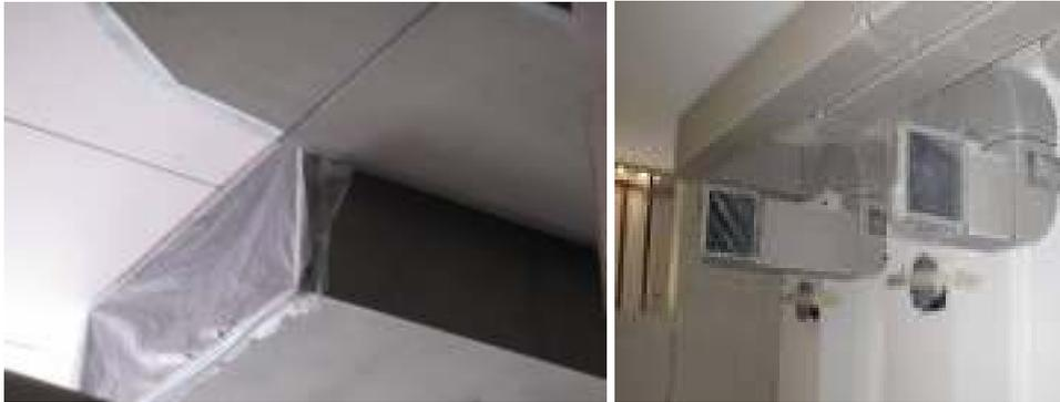
**Figure 3 :** New elementary school of Romarzollo (Arco-Italy)- Covered HVAC ducts in conformance with the IAQ PIndoor Air Quality Management Plan during Construction.
