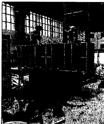
FIG 13. Progressive dumping of earth and its compaction by ramming.
