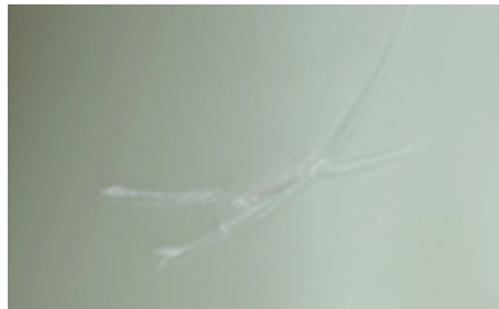
Figure 4: Scratches on the insulation surface
