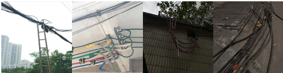
a. Image of slack aging of some wires
